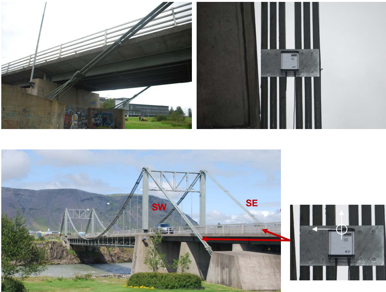
Figure 2: Overview of sensor locations on the bridge.
